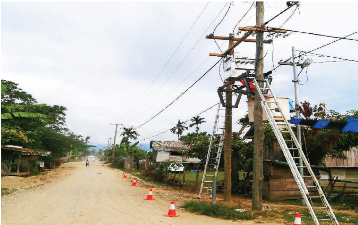
11kV/415V transformer installation
