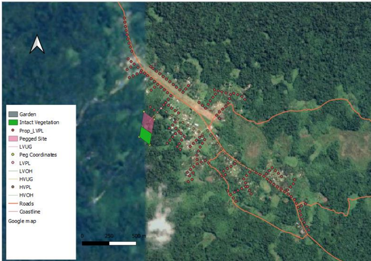
Figure 2: Subproject Site Tingoa.
