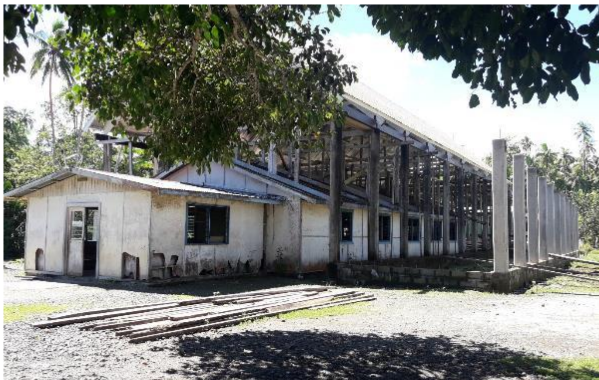
Figure 16: Old SSEC church at Bina village with new structure under construction.
