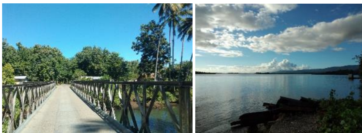
Figure 12: Transportation access-Bina Bridge (left) and Buma Harbor (right).
