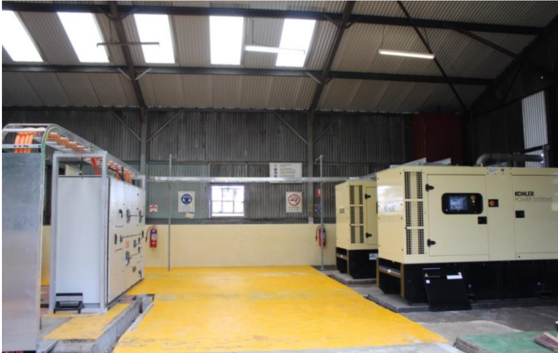
The new-look Tulagi power station
