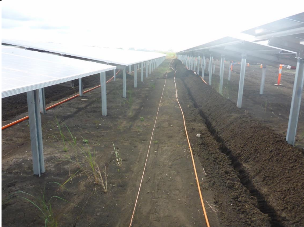
▲ Photo 9 – Installation of solar PV arrays and electrical conduits at Henderson – Fighter 1 solar PV site (2015).
