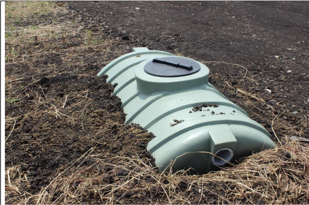
▲ Photo 7 – Installation of septic tank for treating sewage wastes generated from construction and operating staff (2015).
