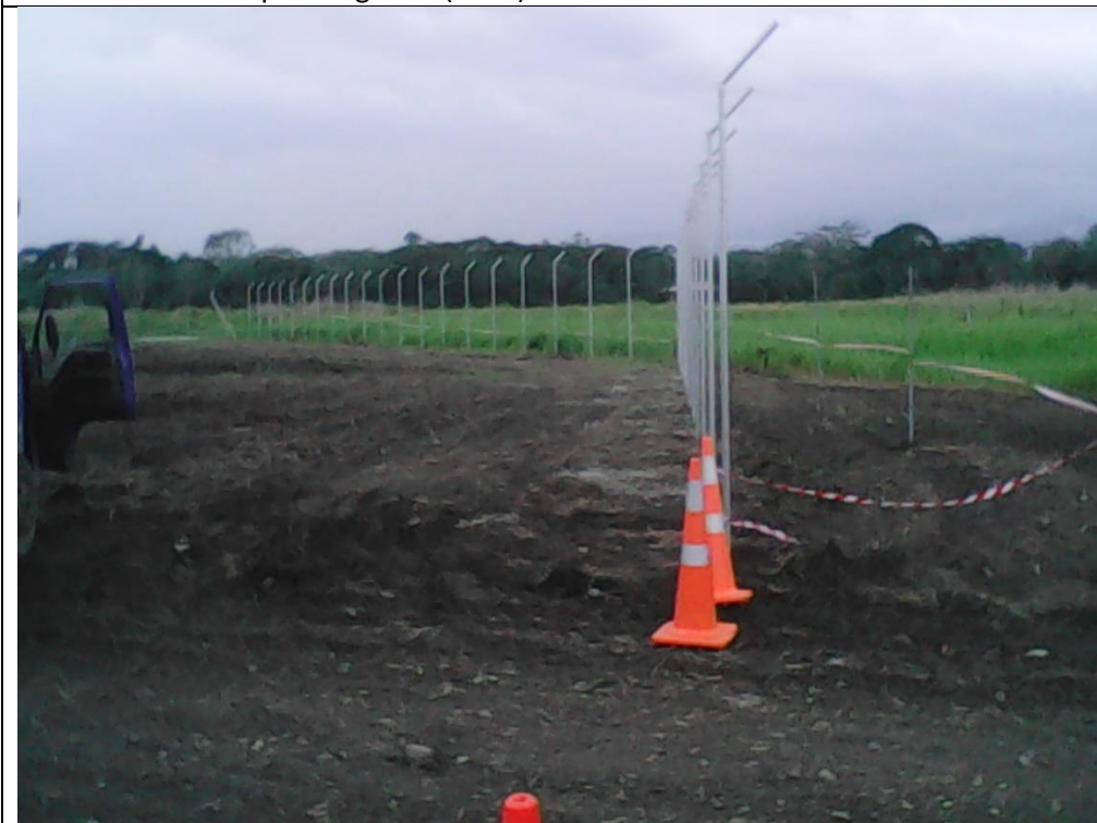
▲ Photo 8 – Installation of chain link security fencing around the perimeter of the Henderson – Fighter 1 solar PV property (2015).
