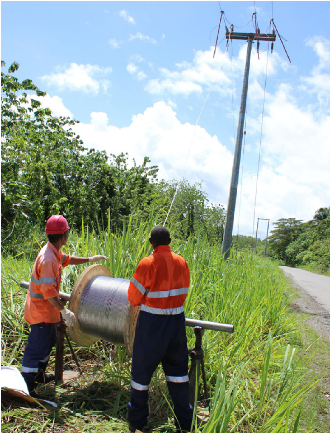
Linesmen pulling the cable through the poles.
