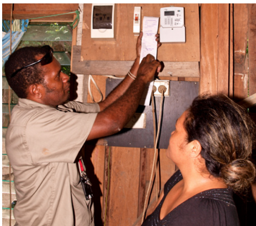
An SIEA technician showing a customer how to use the cash power system after installation.
