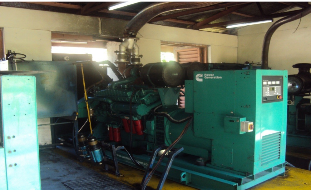
Fig. 1: New 750Kva Cummins Generator Installed at Auki.
