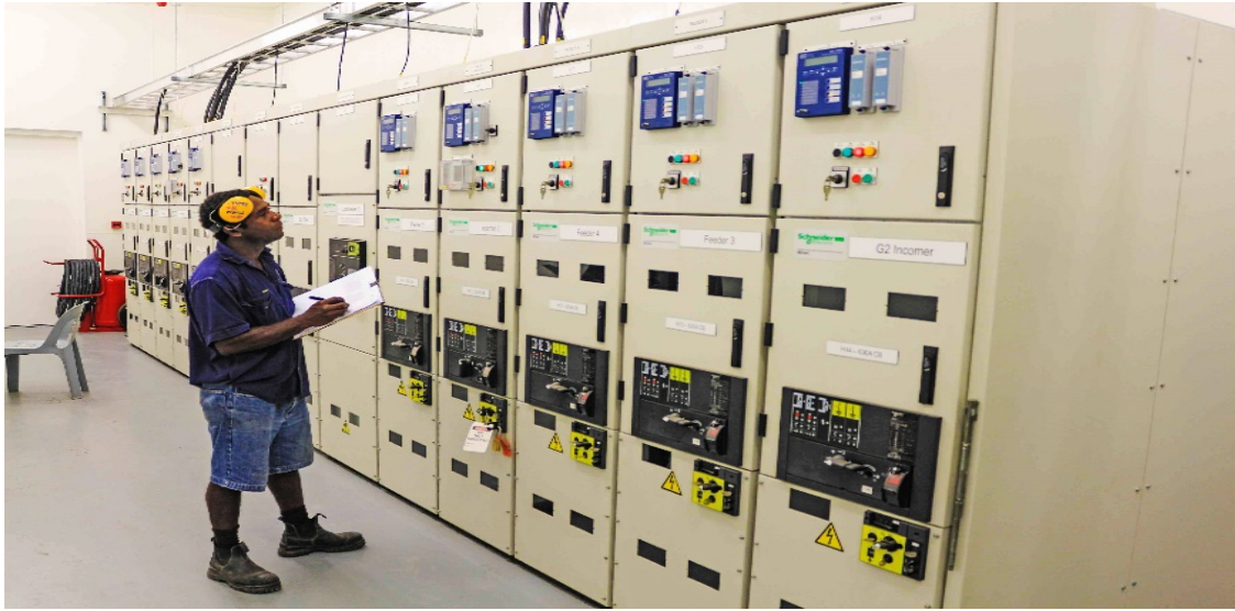
11 kV switchboard at Honiara Power Station
