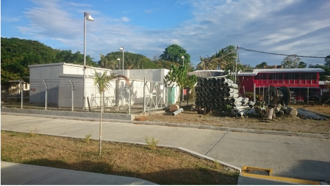
Ranadi Substation before upgrade
