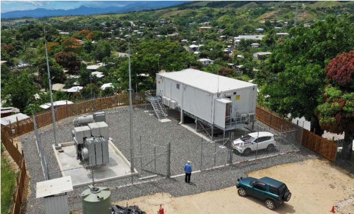
Kola'a Ridge Substation after upgrade
