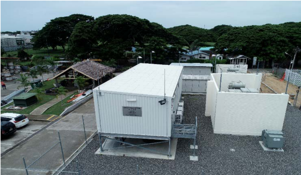
Ranadi Substation after upgrade
