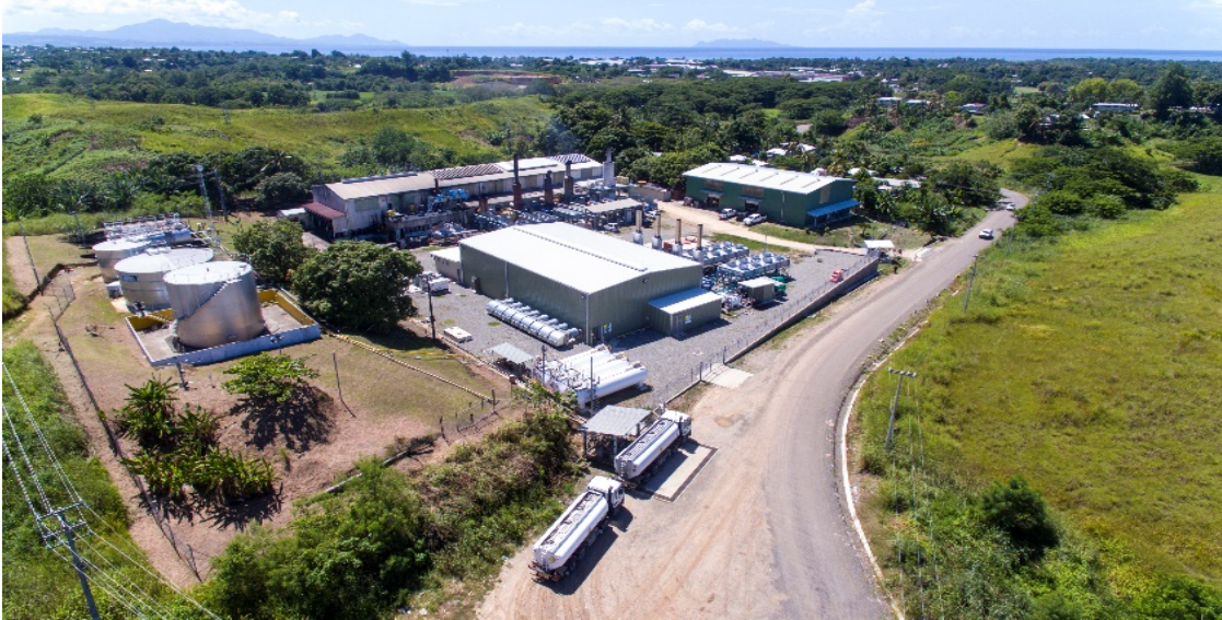
New building housing the 4, 2.5 MW machines- in foreground- Lungga P.S.
